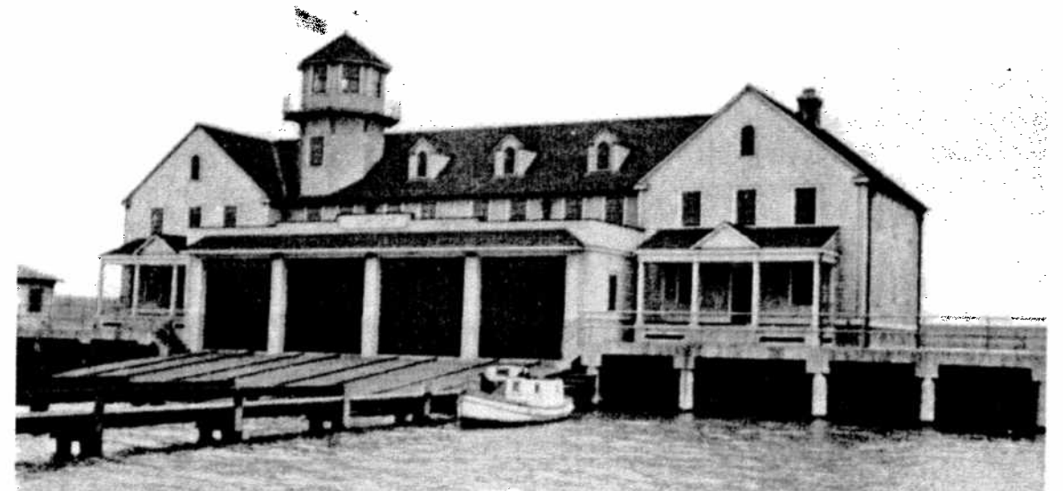
Top: The prior Old Chicago Coast Guard Station (as it had become known) was badly damaged by fire in 1933. It was repaired and put back into service, but was then replaced by the current building in 1936. Bottom: The new station soon after its completion.
